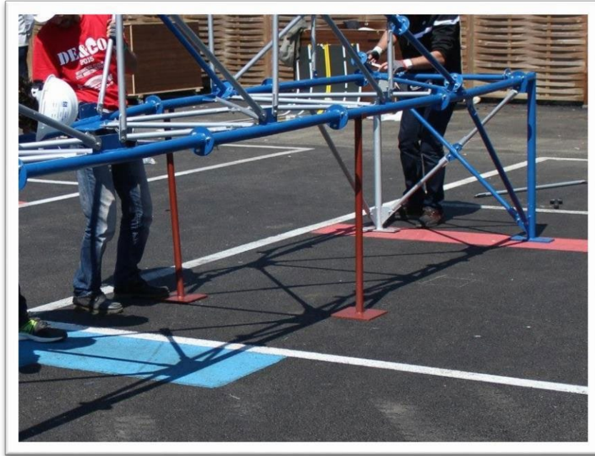
Figure #1: Temporary Support Members (brown painted elements.)
