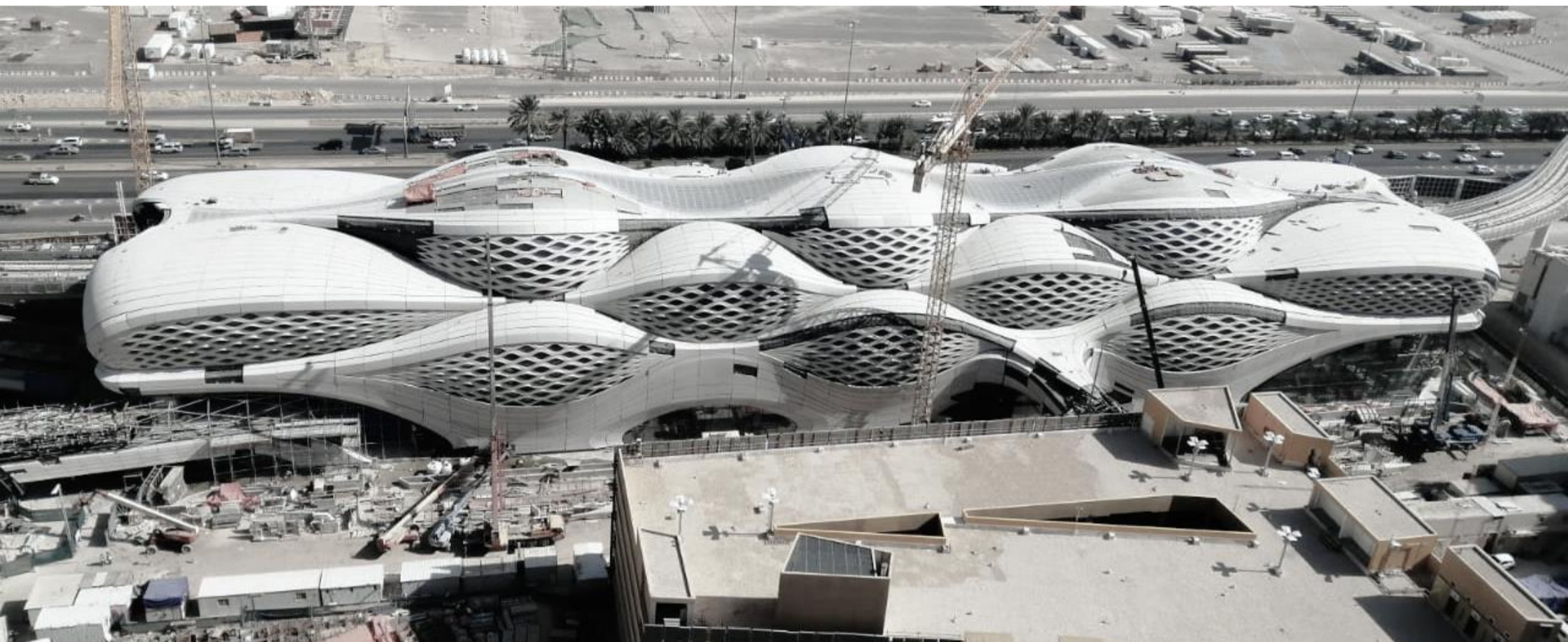
King Abdullah Financial District Metro Station, Riyadh
